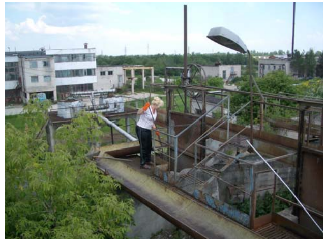
Current wastewater treatment facility in Gatchina. The Programme will help to replace the present manual removal of large solid particles from incoming wastewater with automated technology
