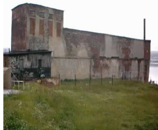
Building No 5 in Andreeva Bay
