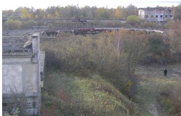
(Above: Overview of the existing facilities with an empty sedimentation tank in the background)
