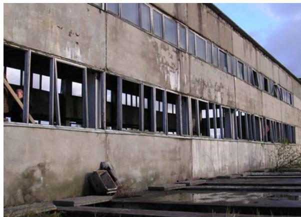
(Above: Present status of the machinery building)
