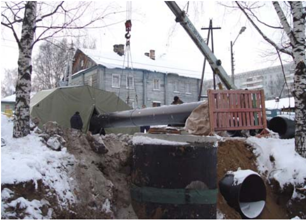
(Above) Construction of the 800mm diameter water main in Syktyvkar
