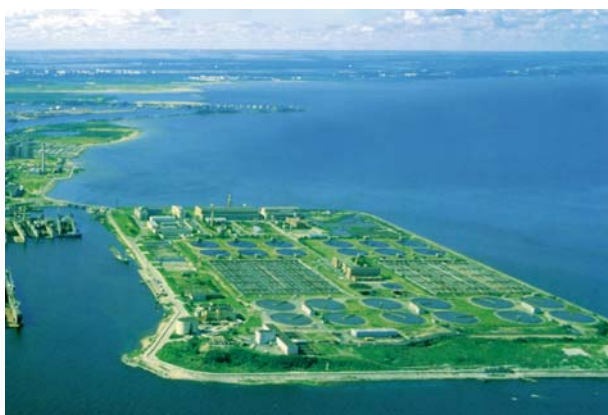
(Above) Overview of the Central Wastewater Treatment Plant located on Bely Island in St Petersburg
