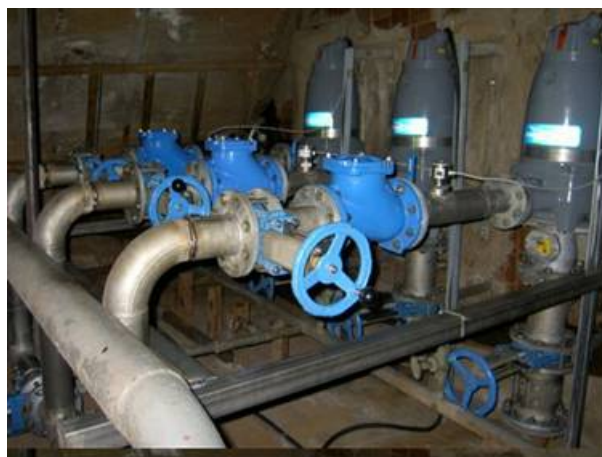
(Above) Rehabilitated sewer pumping stations in Tikhvin
