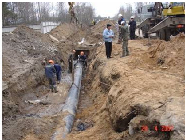
(Above) Construction of a water main in Tikhvin
