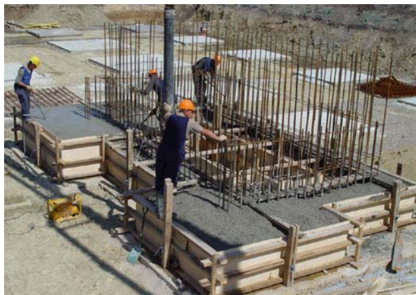
The construction works are running on schedule.
