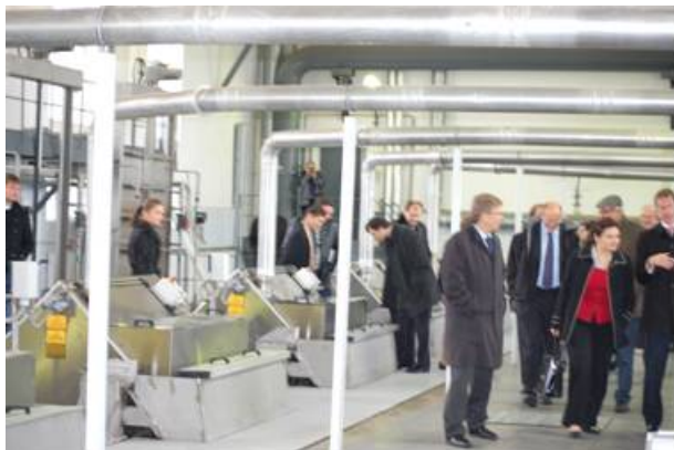
Inside the Northern Wastewater Treatment Plant
