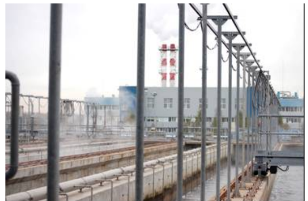
The Northern Wastewater Treatment Plant with the Incinerator plant at the back.
