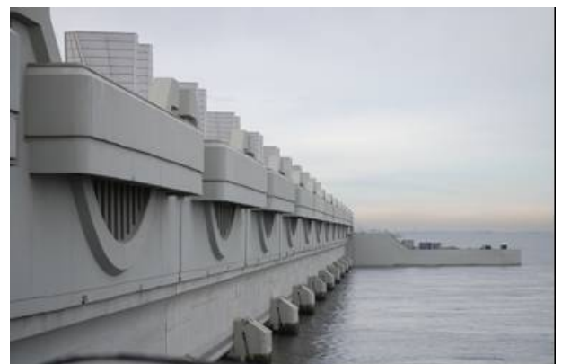
One of the 6 sets of water sluices along the Barrier
