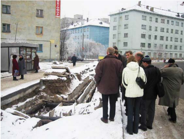
The NDEP's Murmansk District Heating Project will enable the local municipality to modernise the services it provides by replacing corroded heating pipes with pre-insulated, energy-efficient materials.
