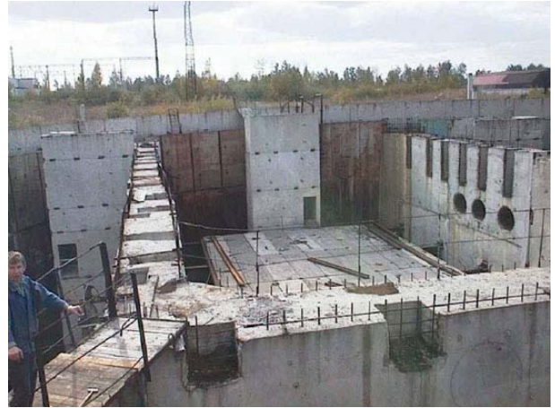
View of the construction site at SWTP
