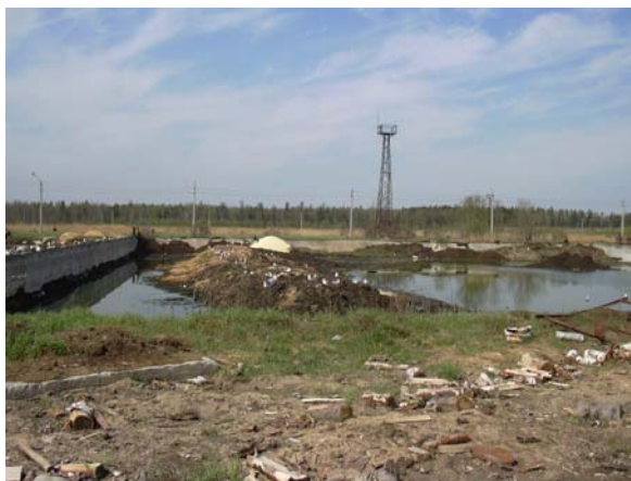
The incinerator will help deal with the waste-water treatment plant's sludge disposal problem
